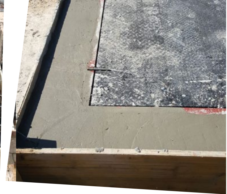
Example of masonry works for weighbridge installation.
